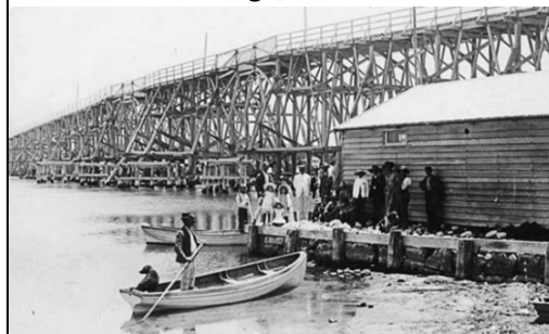
3. Fremantle Bridge, Fremantle
